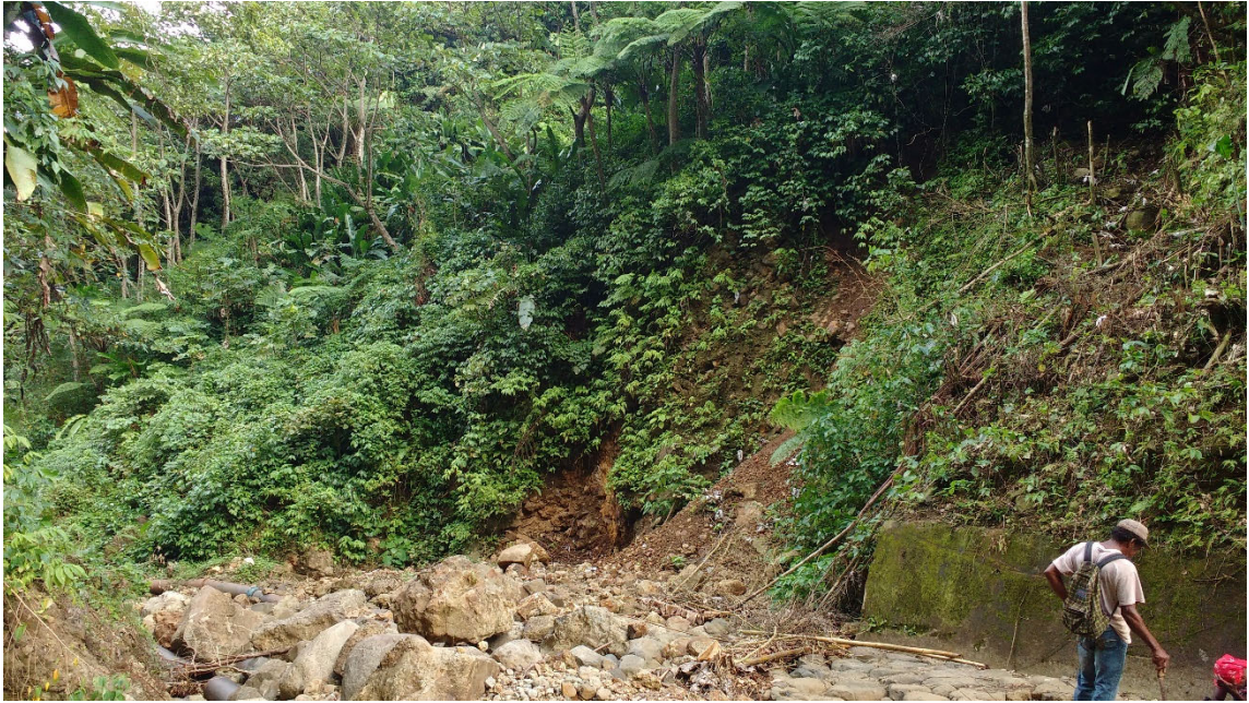
Figure 11: Area below intake along eastern high sloped area that has recently experienced land slippage following heavy rainfall (2018)
