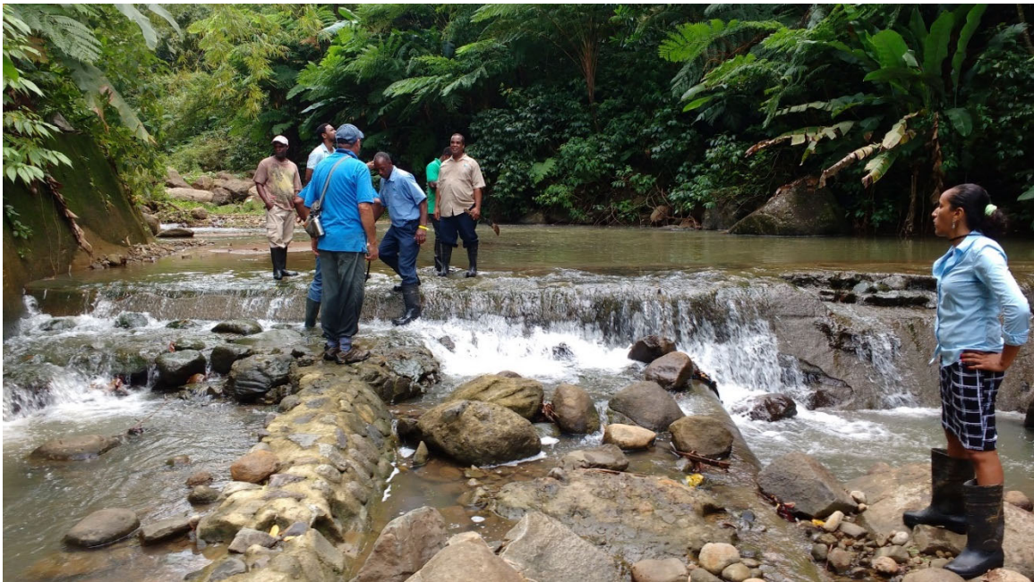
Figure 2: WASCO Intake structure across the flowing Millet River (2017)
