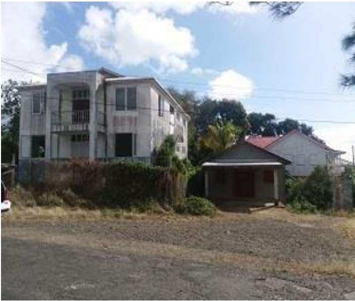
CONSTRUCTION OF THE BLANCHARD COMMUNITY CENTER
