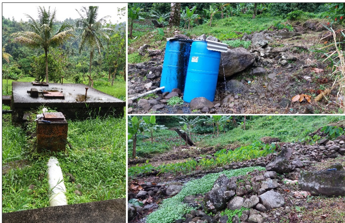
Figure 4.2-1 Water Storage Infrastructure in Fond St. Jacques
