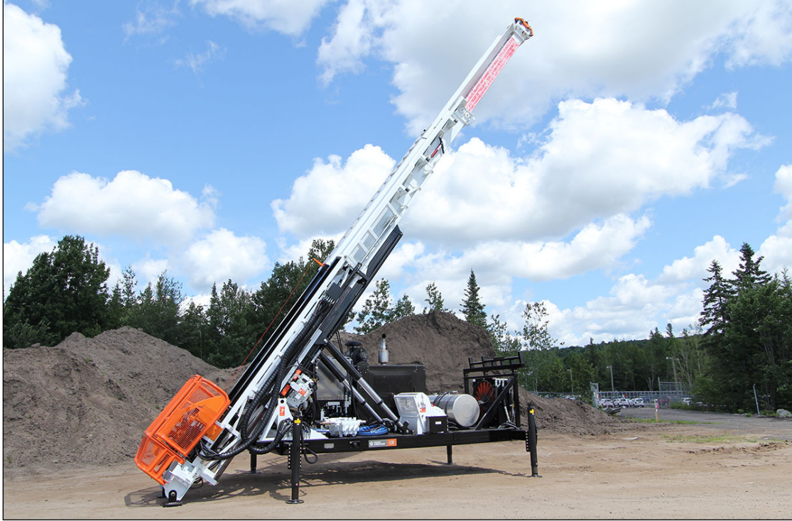
Figure 3.3-4 Example Well Pad and Drill Rig for a Slim-hole Well
