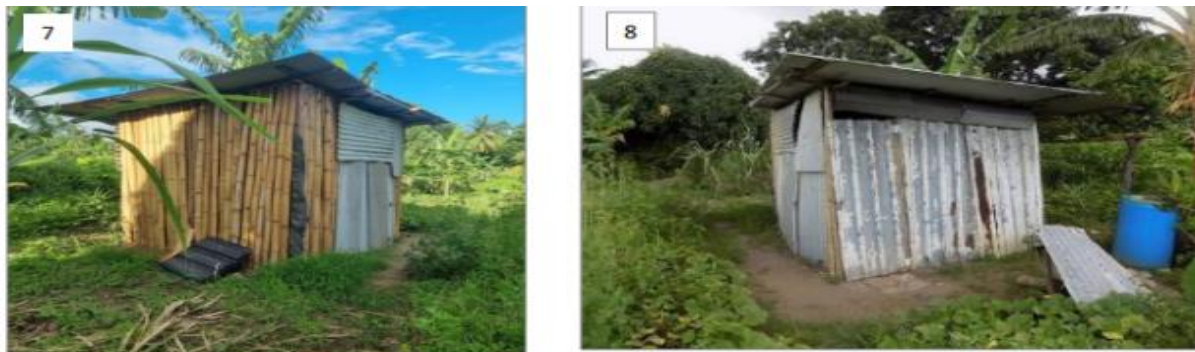
Figure D-2: Material Storage Shed Owner: SPE-03
