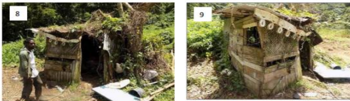
Figure D-3: Material Storage Shed Owner: BLP-01
