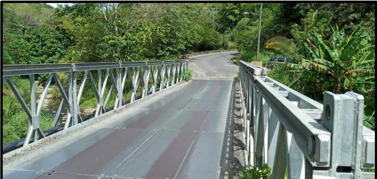
**Figure 7 - Existing Bailey Bridge. Note angled approach from north to enter the bridge.**
