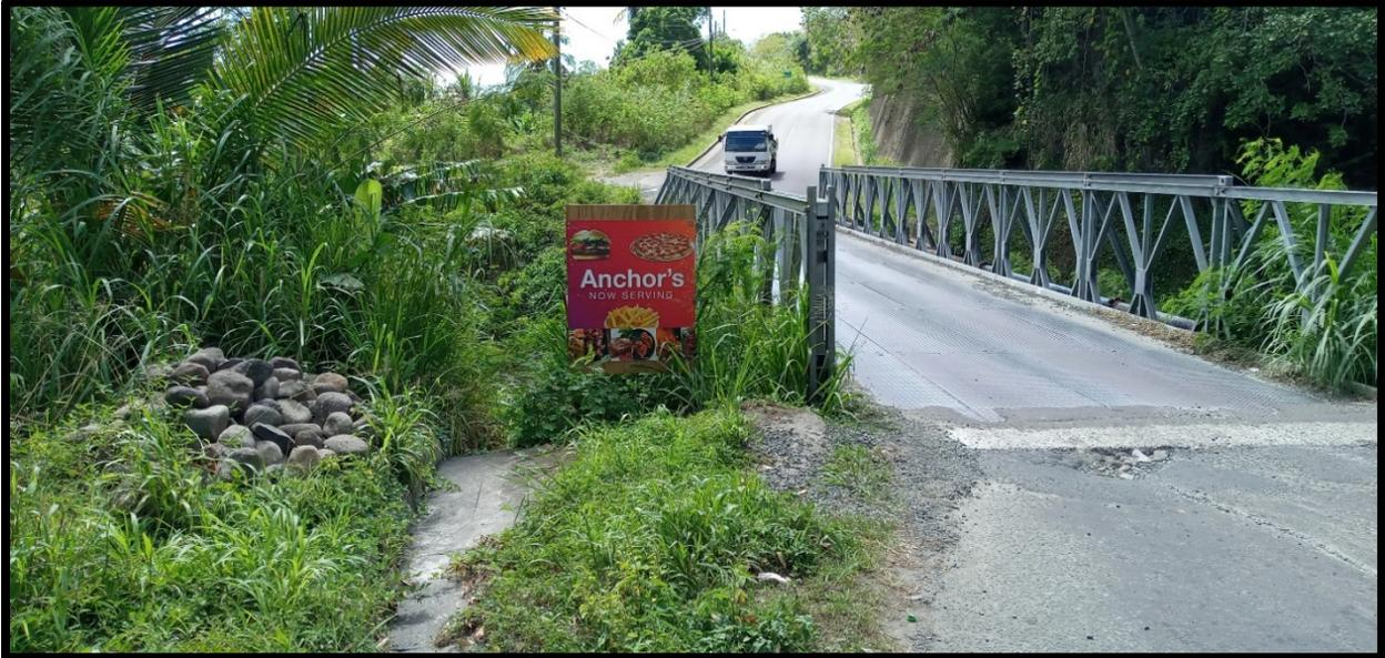
**Figure 6 - Existing Bailey Bridge. Note angled approach of existing road for vehicles to enter the bridge (Looking southward)**
