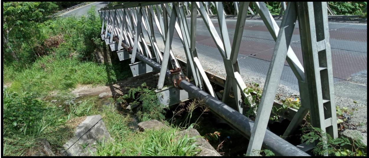
**Figure 5 - WASCO water service line along side of bridge**
